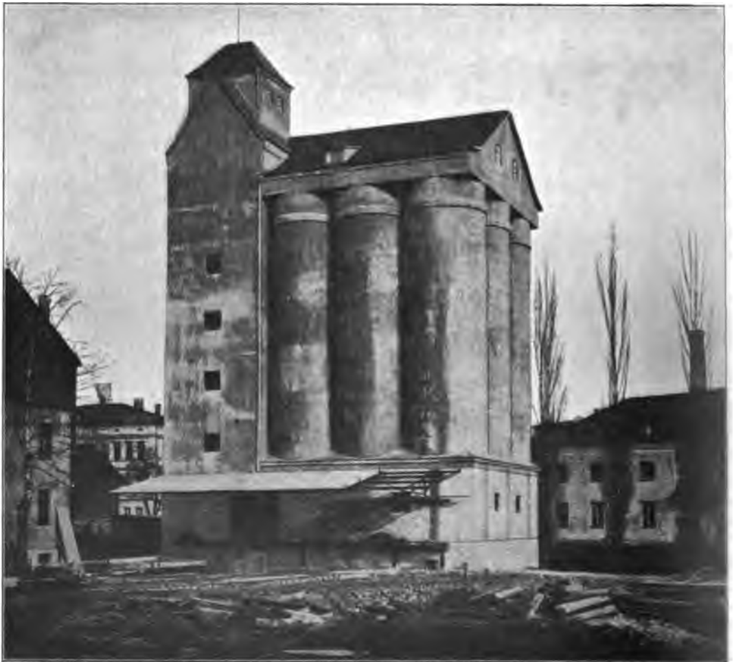
Abb. 106. Silo in Landshut.
